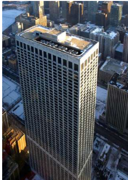
Slika 16. Water Tower Place, Chicago [13]
