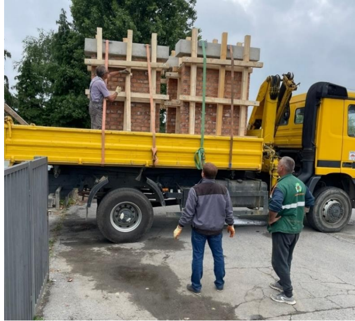
Figure 4.16 Transportation of masonry piers to the laboratory
