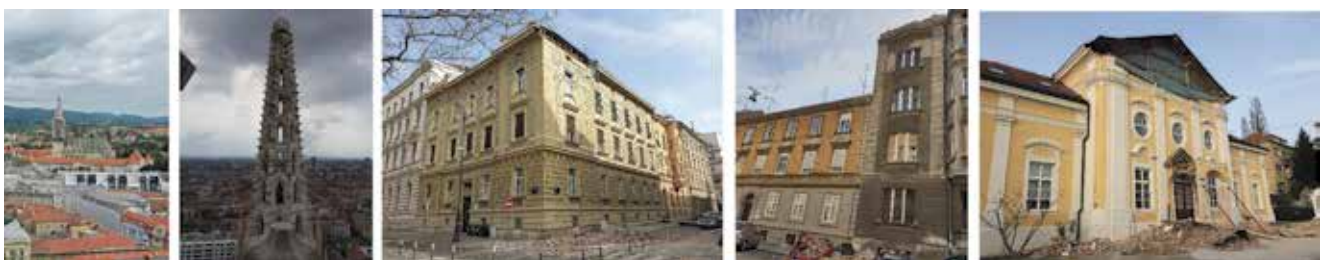
Figure 1. Earthquake effects in historic centre of the city (photos courtesy of: AIR-RMLD d.o.o. www.air-rmld.com, Filip Foretić, Karlo Jandrić)
