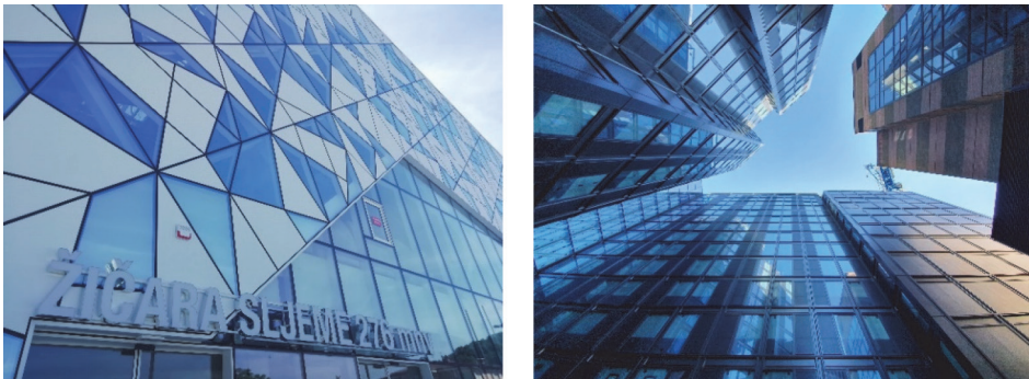
Figure 2. Structural application of aluminium façade systems: a) Cable car Sljeme in Zagreb; b) Urbanest building in London
