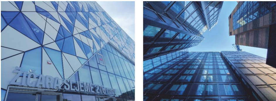
Figure 2. Structural application of aluminium façade systems: a) Cable car Sljeme in Zagreb; b) Urbanest building in London
