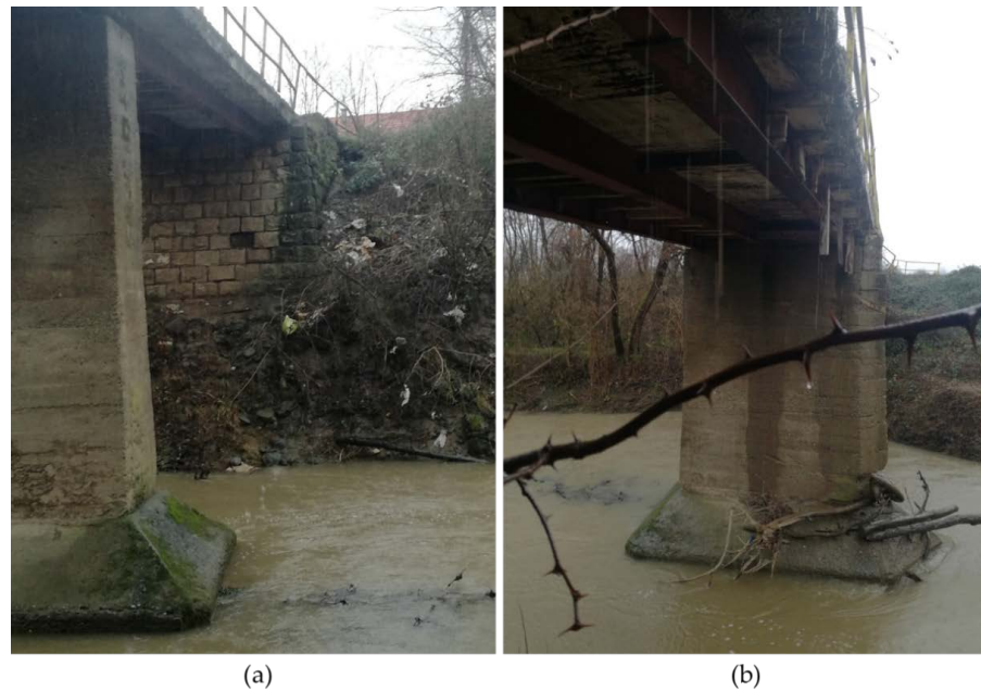
Figure 13. (a) Masonry abutment and (b) composite superstructure of the bridge to Majske Poljane.
