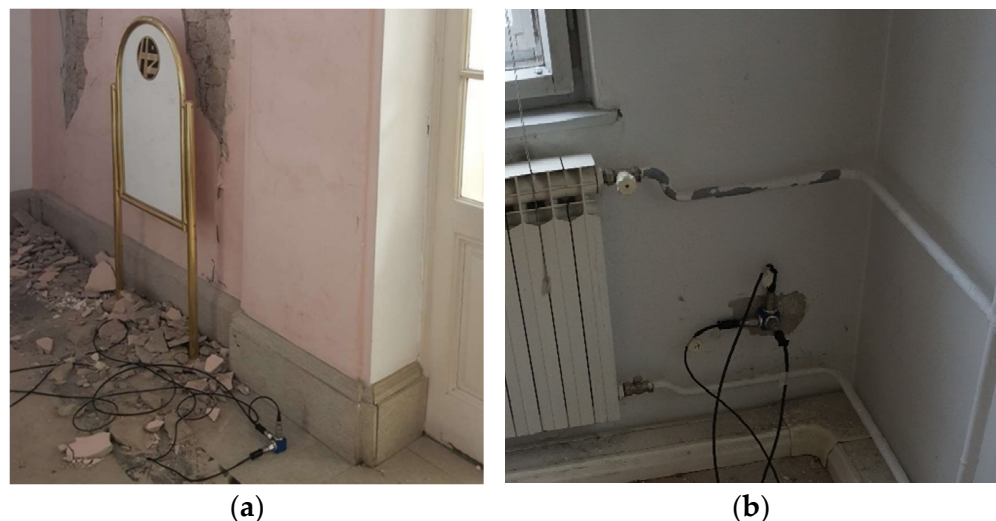
Figure 7. Accelerometer placement on the (a) rigid floor surface and (b) masonry wall structure.
