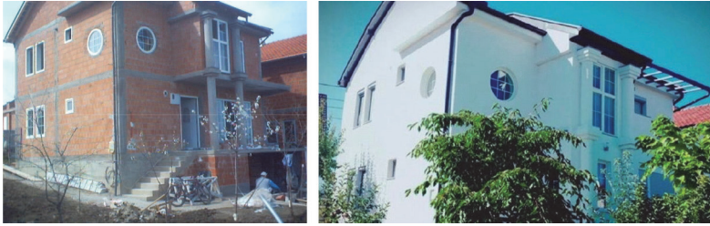
Figure 1. Home of the Qerimi family before and after the intervention [24]
