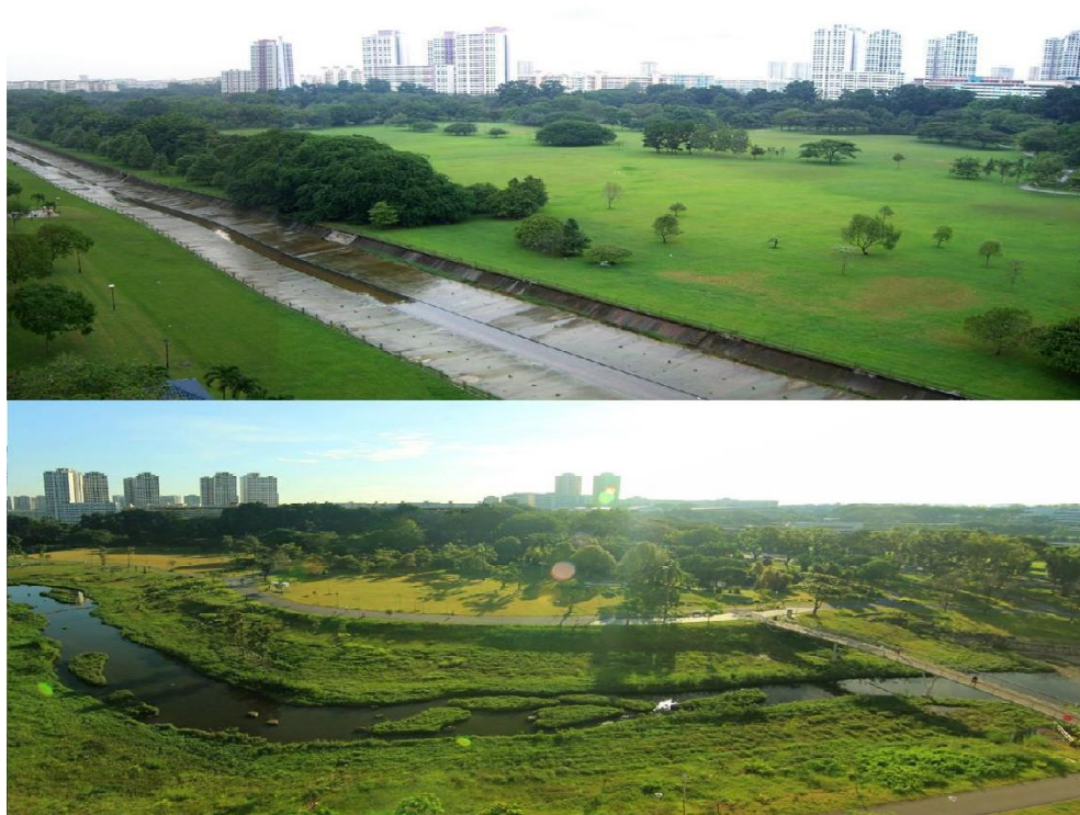
Figure 2: The Kallang canal before and after the intervention (World Architecture News, 2021)
