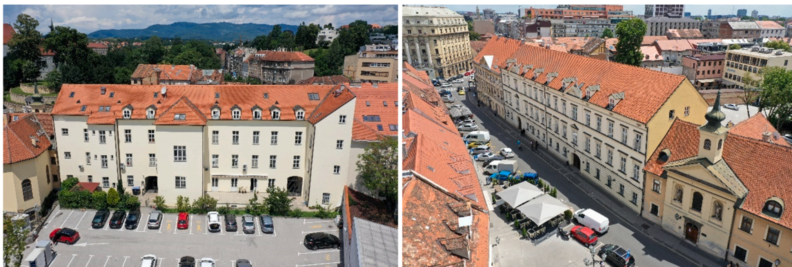
Fig. 3. South and north façade of the case study building.
