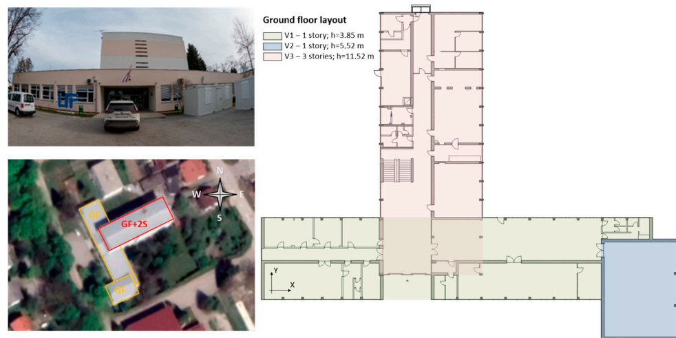
Figure 3. Case study building.
