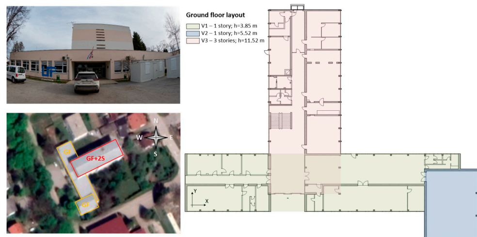
Figure 3. Case study building.
