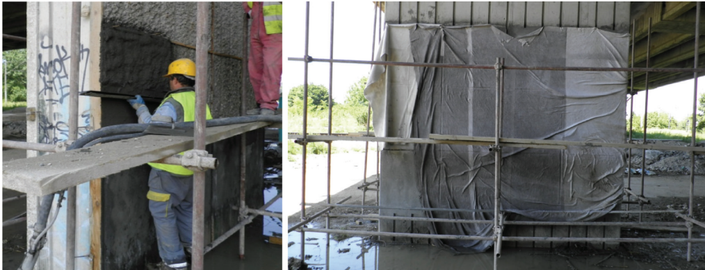
Fig. 3: Finishing of repair mortar surface (left) and curing of repair mortar (right).
