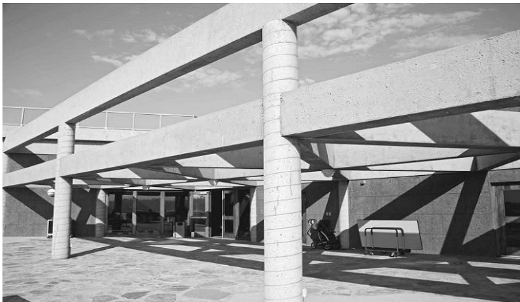
Slika 1.4. Prikaz statički neodređenog nosača (Izvor: [ https://theconstructor.org/structural-engg/analysis/determinate-and-indeterminate-structures/3483/ ])
