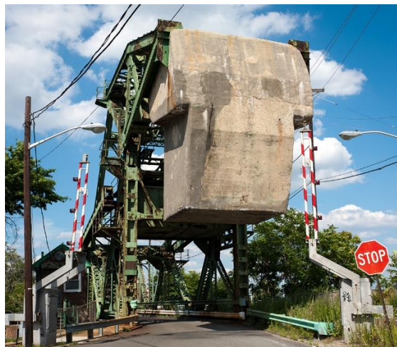
Slika 20.: Protuuteg South Front Street bridge-a [19]
