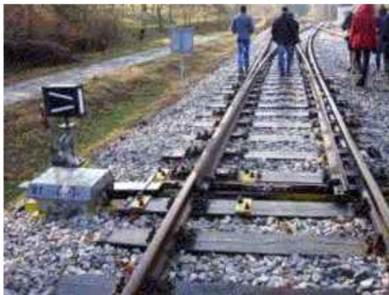
Figure 3 Disconnector switch on special track
