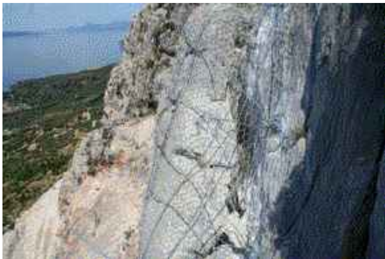
Figure 7 Retaining unstable boulders
