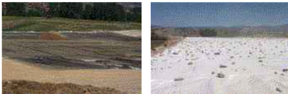
Figure 9 The geogrids were placed over the full embankment width, starting at app. 373 m altitude, which is approx. 0.5 m above the 100–year flood level. A combigrid was installed underneath the road base course over a width of approx 30.9 m. A combigrid was installed transversely to the road axis, with an overlapping of a min 300 mm in both adjacent and longitudinal directions.
