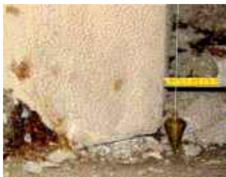
Figure 2 Vertical impairment and deviation of bearings
