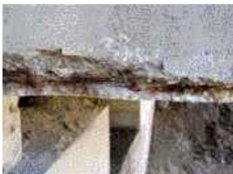
Figure 3 Exposed, corroded reinforcement
