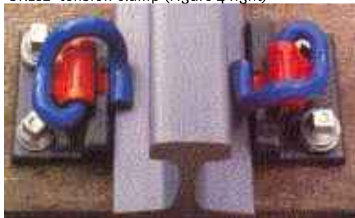
Figure 4 Resilient rail fastening for wooden sleepers
