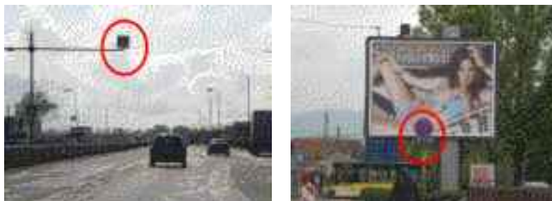
Figure 7 Information does not grab road users attention (driver does not see the pedestrian crossing, no zebra marking, road layout is not appropriate and the sign is not visible enough)
