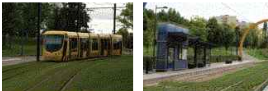
Figure 5 Perfect green track (left) in Mulhouse and the damaged green track at a terminal stop (right) caused by (too) long idle time and multiple mechanical impacts by trespassing passengers
