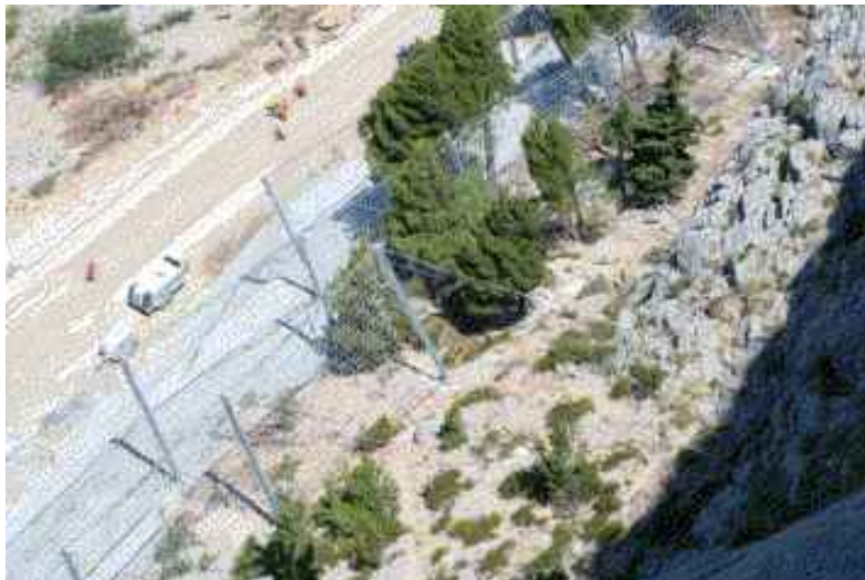
Figure 6 Constructed barriers Retaining unstable boulders
