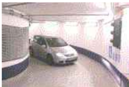
Figure 7 Spiral ramp 4 m in width, inner radius 4,75 m (My Zeil, Frankfurt)
