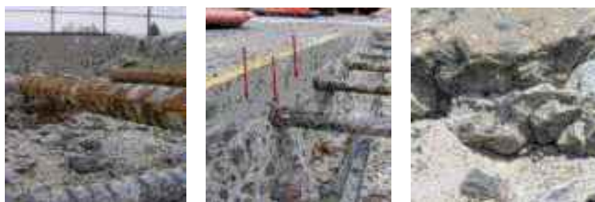
Figure 1 Rebar corrosion, delamination and concrete degradation.
