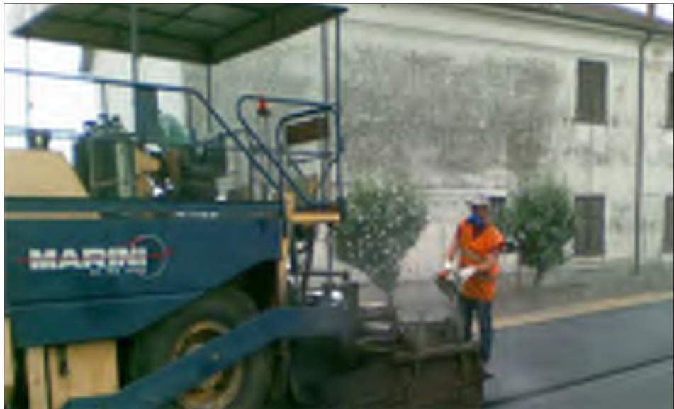
Figure 9 Laying of the wearing course
