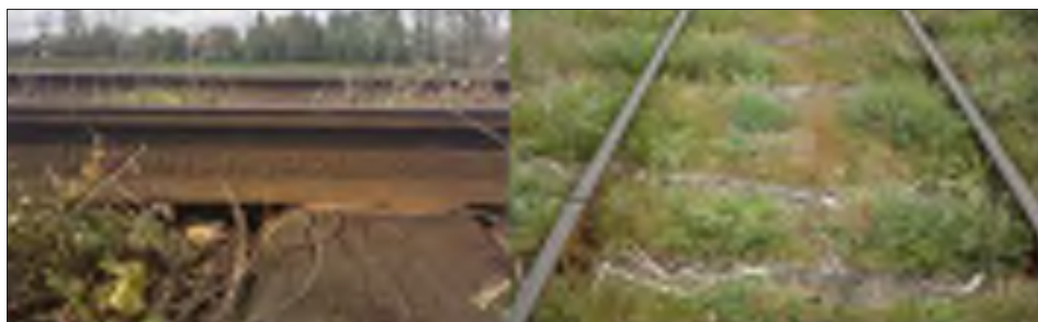
Figure 2 Track on the existing railway line Subotica (Freight) – Horgos – Serbian Hungarian border [1]
