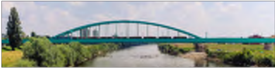
Figure 3 Static testing of the bridge “Sava” – two compositions in the main span
