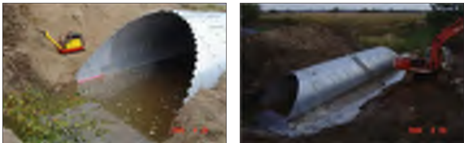
Figure 3 Initial phases of the construction of the structure in a watercourse
