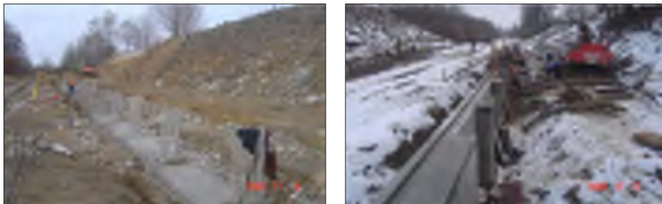
Figure 7 Supporting the soil-steel structure on a wall topping the piles
