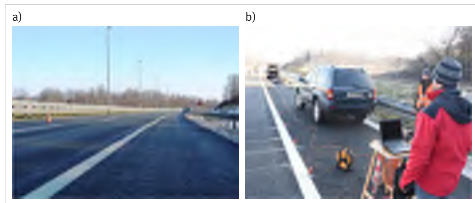
Figure 7 a) Pavement bulging in 9.5 th km, b) seismic data acquisition
