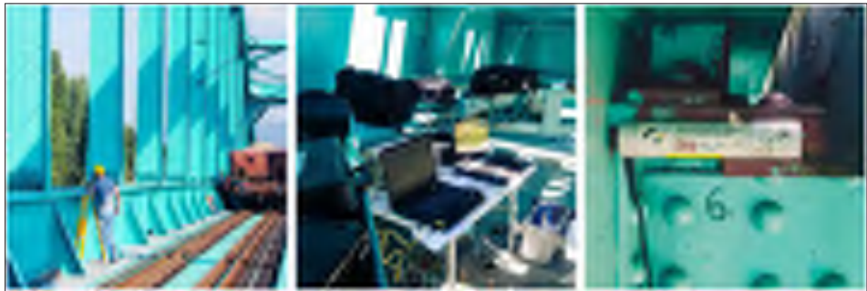
Figure 4 Vertical displacement measurement (left), data acquisition system (middle) and strain measurement sensor (right) on bridge “Sava”
