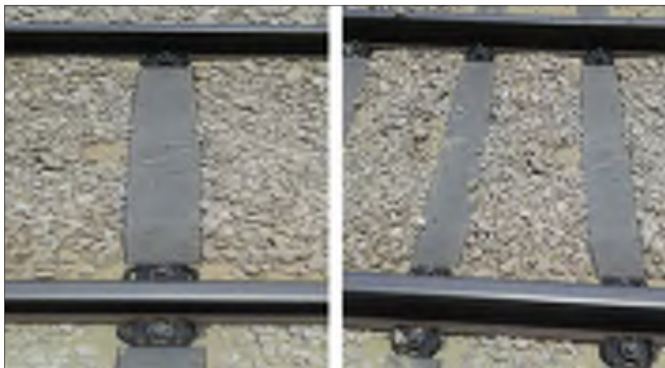
Figure 3 New Installed concrete sleepers (see table 6 mix design)
