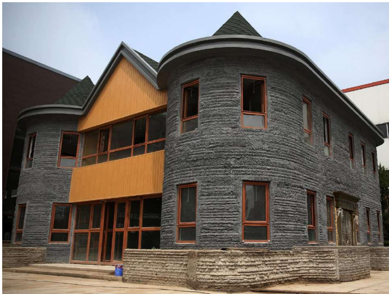
Slika 4 3D ispisana kuća u Kini, 2016 ( https://www.realestate.com.au/news/totally-3d-printed-house-created-in-china-over-45-days/ )
