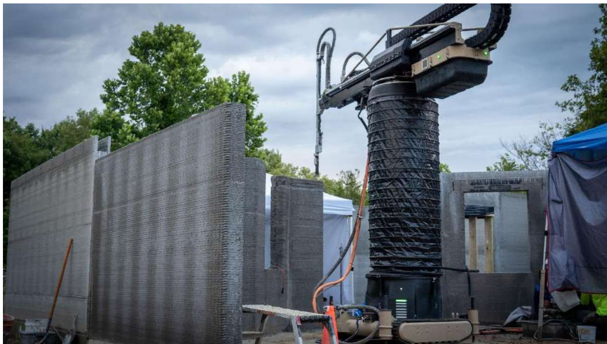
Slika 13 Sistem kрана na gradilištu ( https://blog.apis-cor.com/the-effects-of-cement-and-global-warming-0 )
