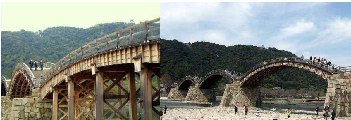
Slike 10. i 11. Most Kintai ( https://www.atlasobscura.com/places/kintai-bridge )
