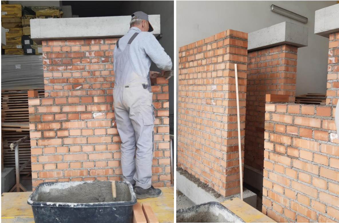
Figure 4.3 Construction process of the masonry piers
