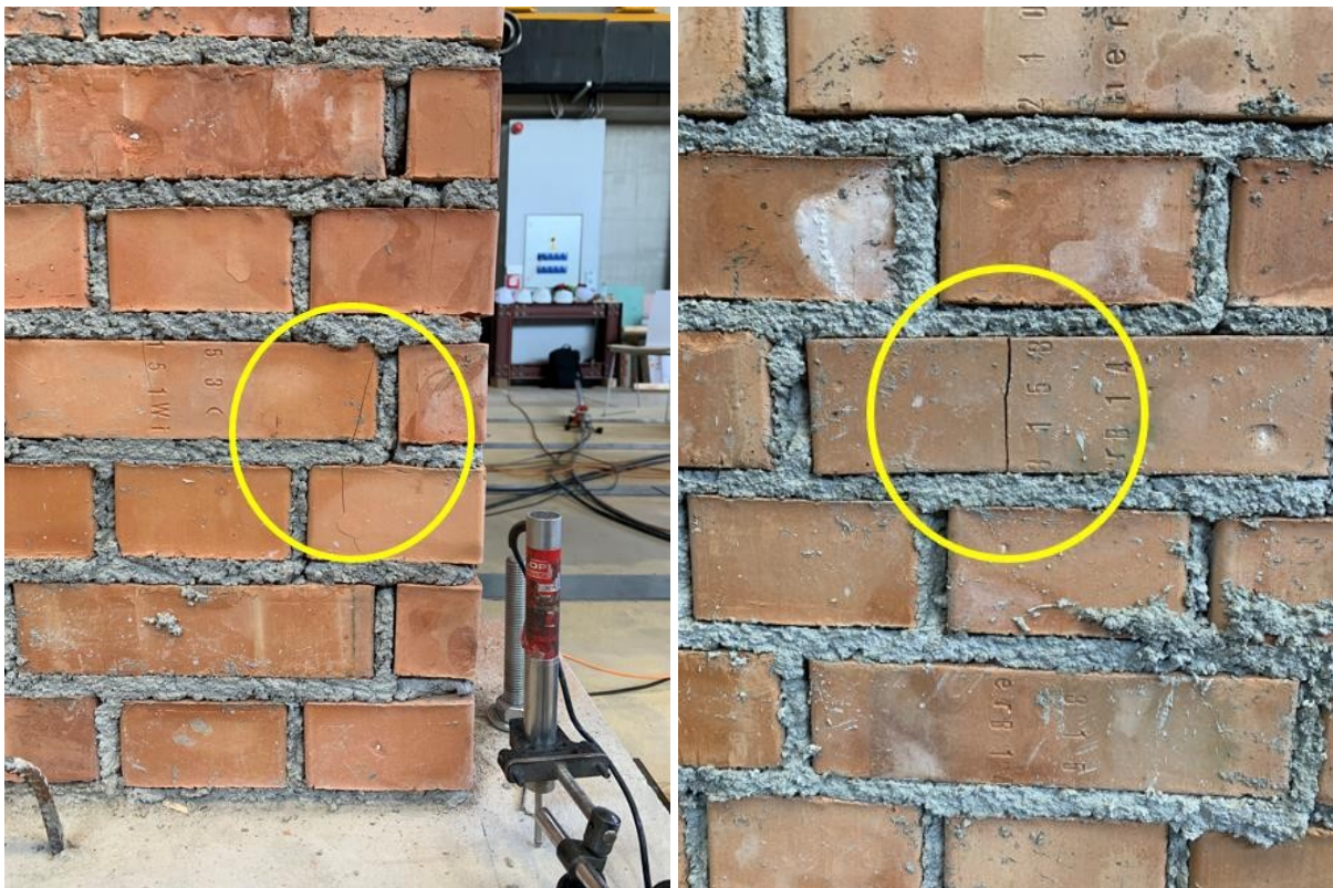
Figure 4.22 First and second crack of URM 1 pier
