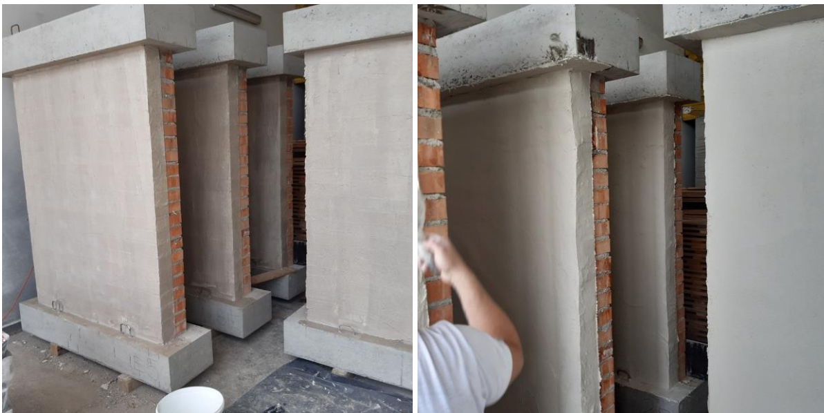
Figure 4.7 Strengthened masonry piers
