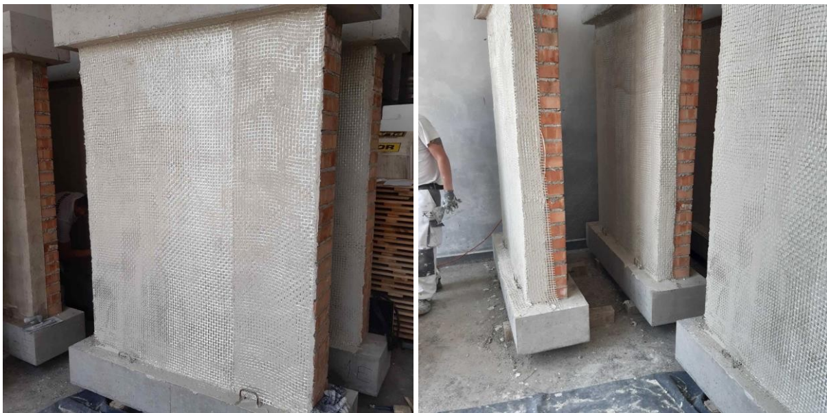
Figure 4.5 Application of the glass fibre mesh
