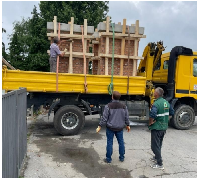
Figure 4.16 Transportation of masonry piers to the laboratory
