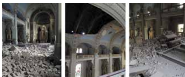
Figure 33. Damage to Basilica of the Sacred Heart of Jesus (photos courtesy of: Ivan Ćurić)
