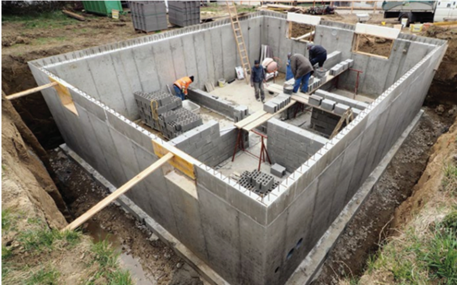
Figure 3. Commercial rigid basement construction
