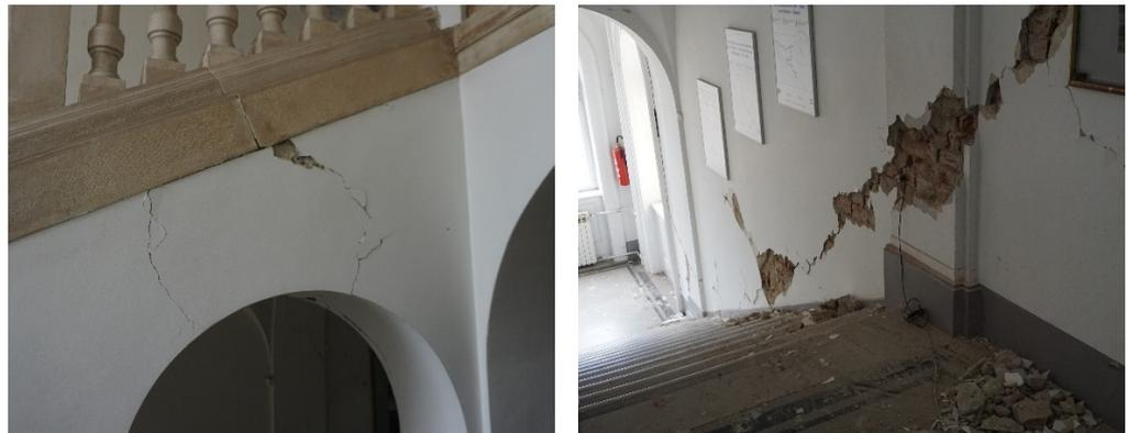
**Figure 4.** Damage to the central staircase in the HŽI head-office building.
