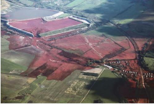
Figure 1. Red mud landfill [9]
