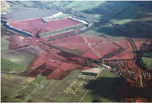
Figure 1. Red mud landfill [9]
