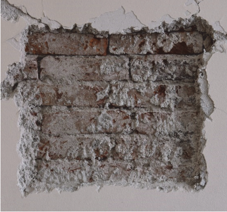
Figure 6. Masonry wall – Catholic Faculty of Theology
