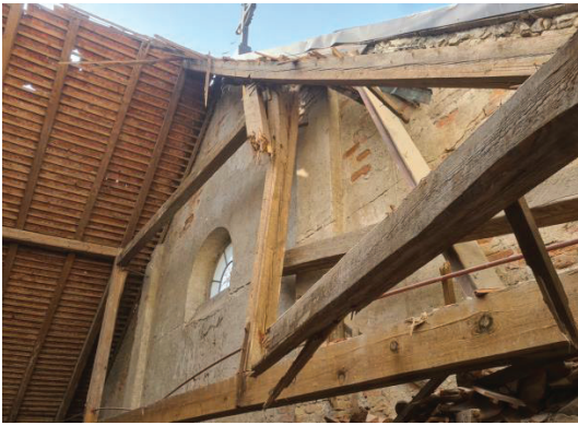
Figure 6: Timber roof collapse – Sisak cathedral (photo credit: Studio Arhing d.o.o.)
