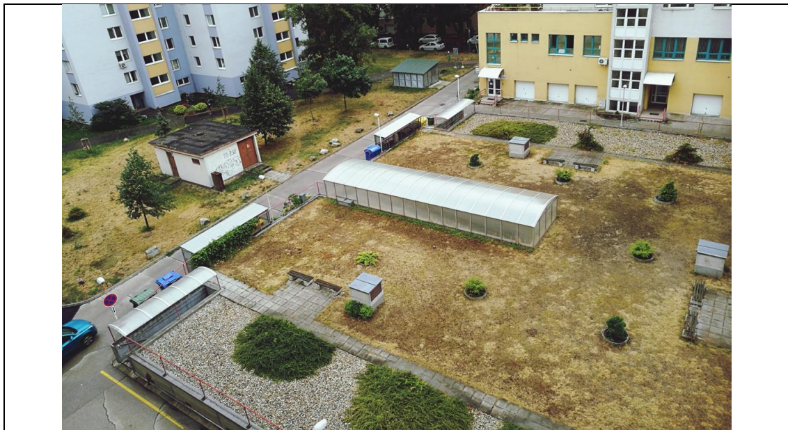
Fig. 2: Top view of the green garage roof
