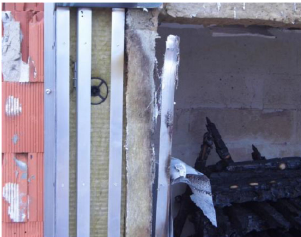
Figure 6. Sample 2- influence of vertical barrier on fire spread.
