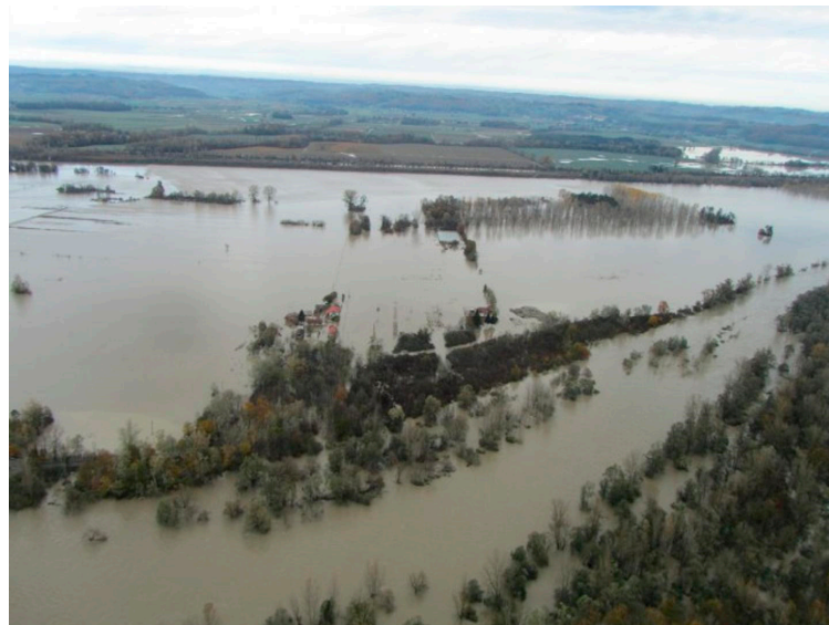
Figure 2. Flood area after breaching Otok Virje-Brezje levee [34].
