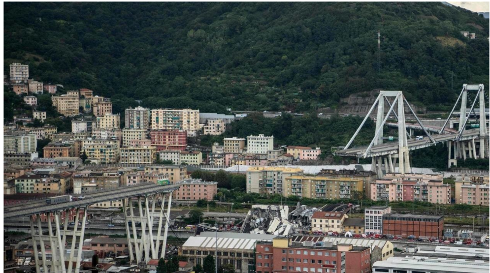
Figure 1. View of the collapsed part of the Polcever viaduct in Genoa, August 2018. (AP Photo, Antonio Calanni, 2018).
