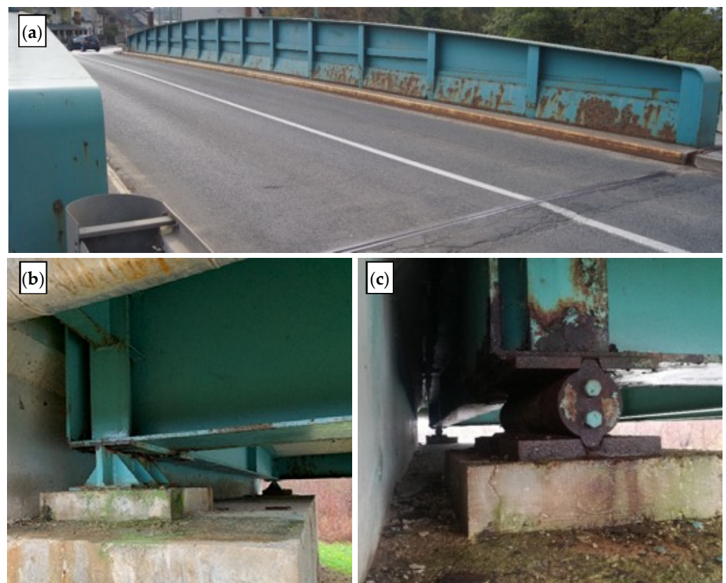
Figure 7. Glina bridge: (a) main girder and carriageway; (b) fixed bearing; (c) movable bearing.
