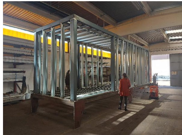
Figure 5. Load bearing steel structure of the MUZA: left —numerical model, right —realized structure.
