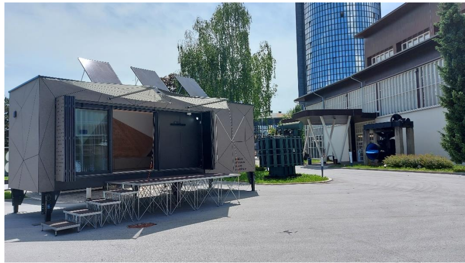
Figure 4. View of the main façade of the MUZA constructed with the LSF system.
