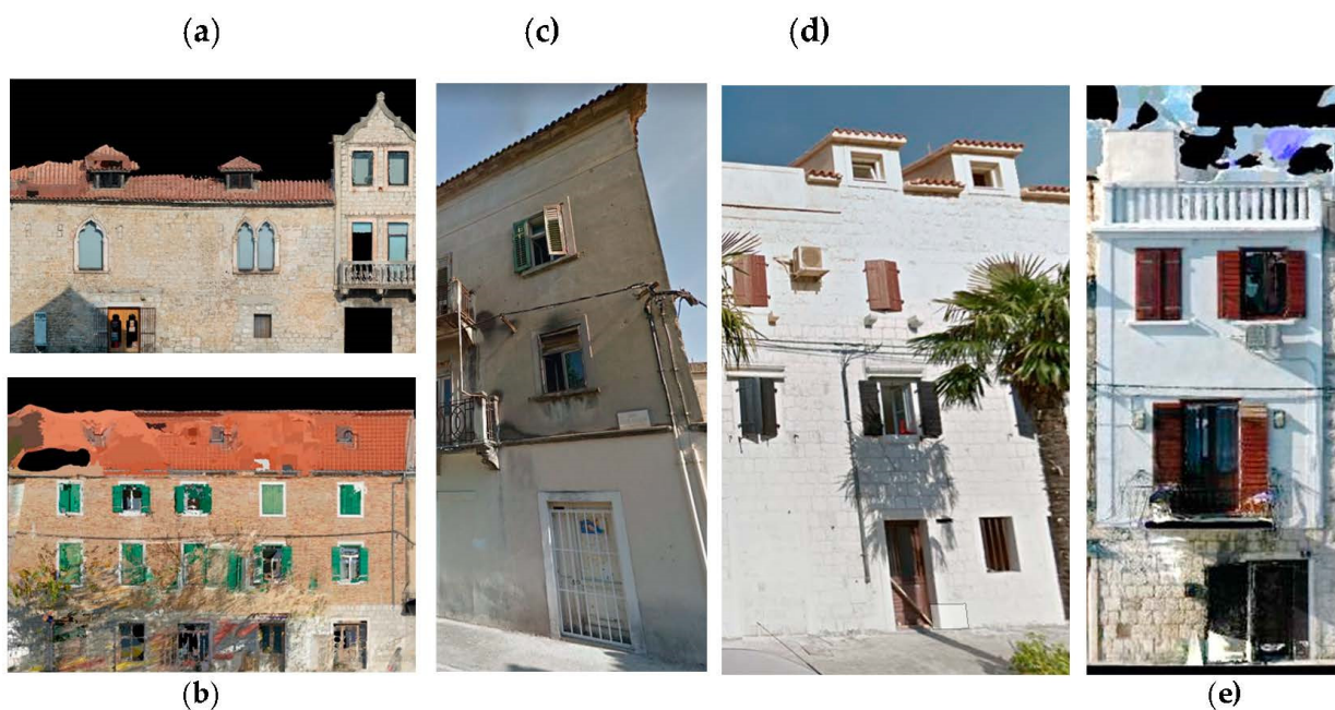
Figure 8. Selected five buildings for the Kaštela study area. Elevations photographed or reconstructed by photogrammetry.
