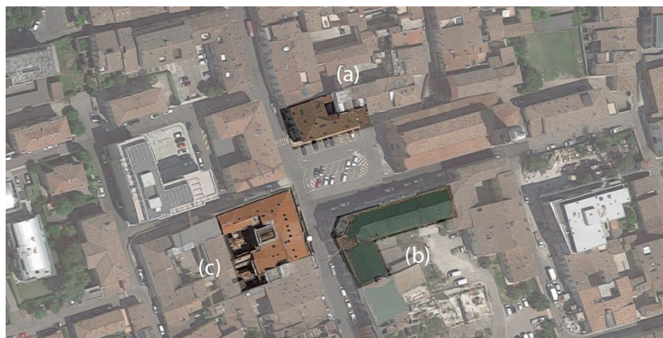
Figure 5. A view of the Mirandola case study site and the three buildings analysed.
