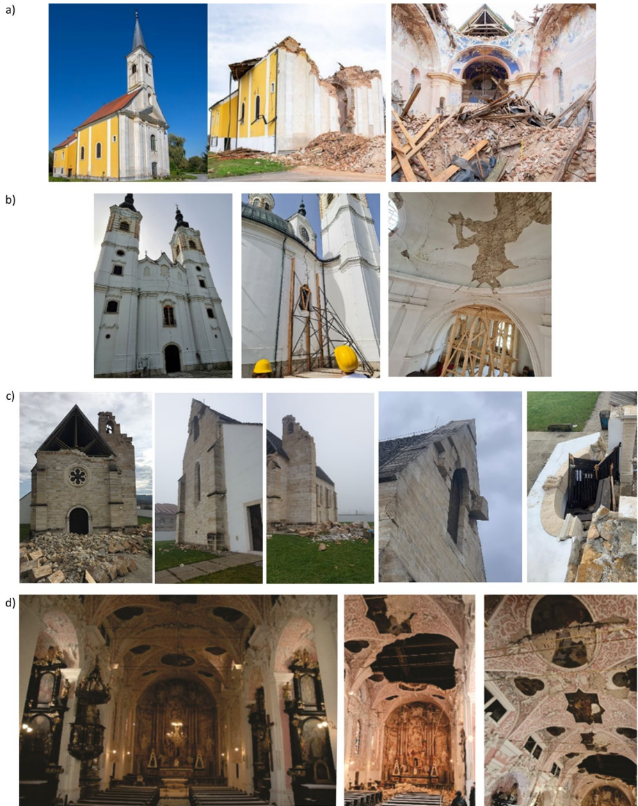
Fig. 14 Damage to sacral buildings: a Church of St. Nicholas and St. Vid in Žažina, b Church of St. Mary Magdalene in Sela, c Church of the Assumption of the Virgin Mary in Gora, and d Church of St. Catherine in Zagreb after Zagreb earthquake (left) and after Petrinja earthquake (center and right) (photos: courtesy of Sisak archdiocese 2021; CCEE 2022; and Martina Vujanović, 2022)
