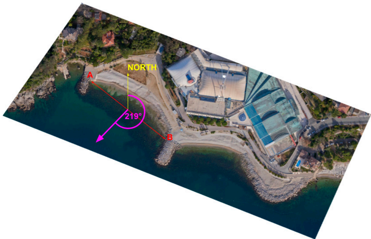
Figure A3. Aerial picture of Ploče beach showing a red line connecting end points (A and B) of the western beach cell, a yellow arrow pointing north, and a purple arrow perpendicular to the red line connecting beach endpoints (A and B) and in the direction of the beach orientation, which closes an angle of 219^\circ from north.
