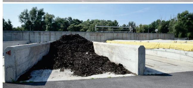
Figure 5 Constructed composting plant within WWTP Varazdin
