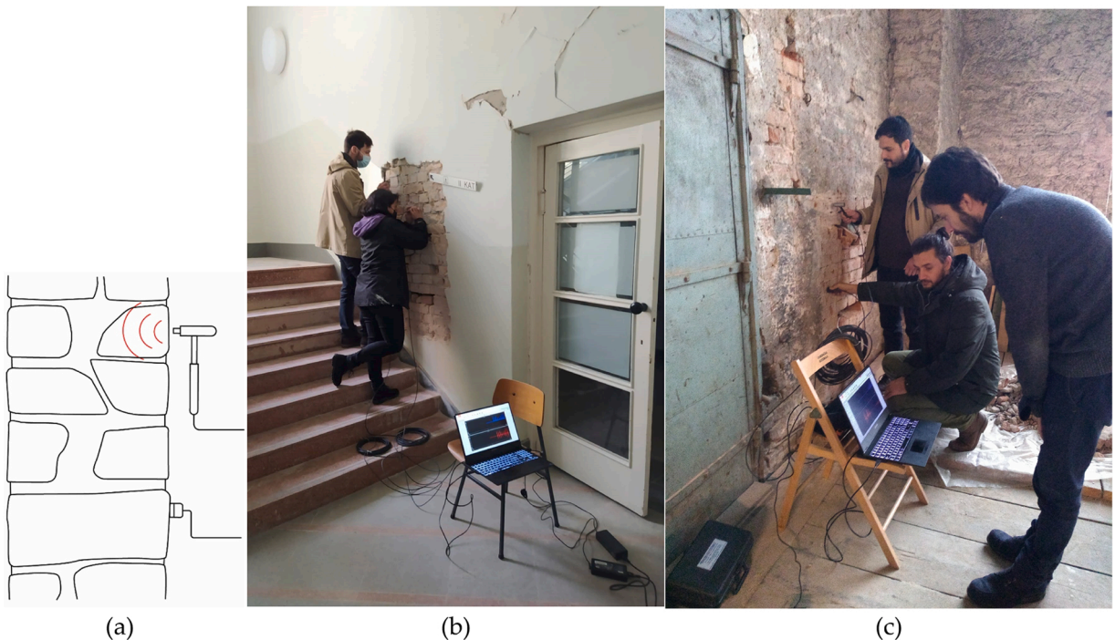
Fig. 4. (a) Typical indirect sonic test transmission method; and (b,c) on-site application of sonic tests.
