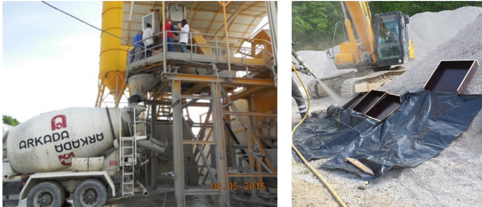
Fig. 4. Spraying equipment and spraying procedure.
