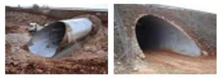
Figure 9 Installation of animal underpass – phase II and animal underpass in km 5+030,00 of Adriatic Highway – ISTRIAN "Y"
