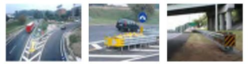
Figure 6 Safe barrier systems with proper ends
