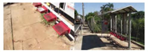
Figure 3 Examples of regularized sidewalks with curbside cutouts for easy access to people with reduced mobility, however, with the absence of elevated curbside to facilitate boarding of wheelchair users
