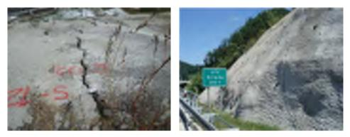
Figure 2 Defects and crack on Straža jug cut
