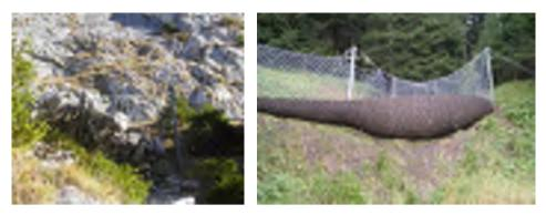
Figure 1 Snow net barrier loaded with rockfall (left), rockfall barrier loaded with a shallow landslide (right)
