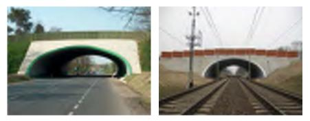
Figure 5 Animal overpass in Trzebaw (2002) (span of 17,68m) and above railway, Rzepin (2008); Poland
