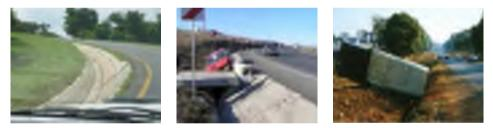
Figure 3 Unsafe drainage structures
