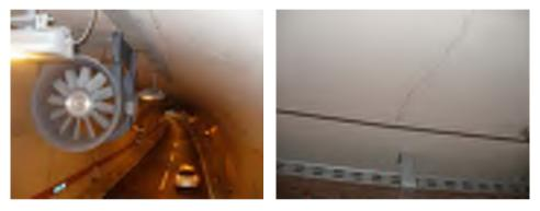
Figure 1 Crack in secondary concrete tunnel lining
