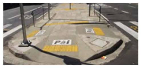
Figure 8 Ramps to facilitate access of persons with disabilities or reduced mobility
