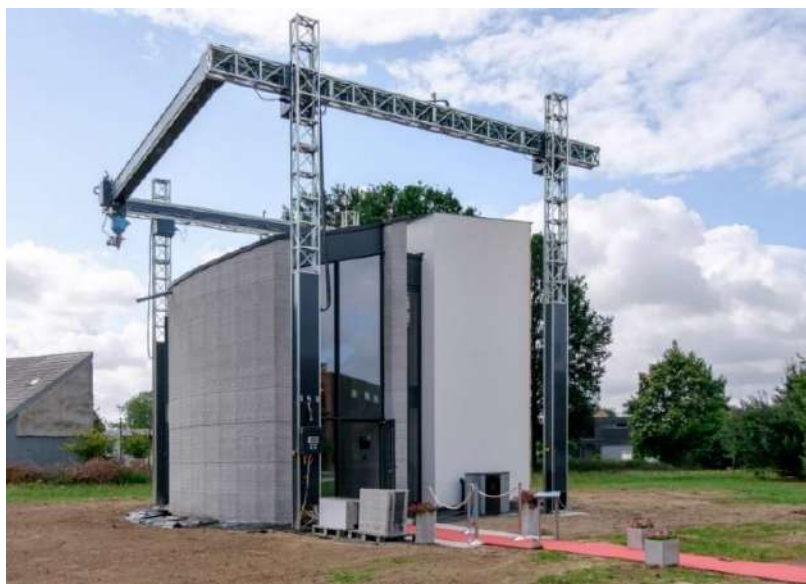
Slika 12 Gantry sistem gradnje na gradilištu ( https://www.re-thinkingthefuture.com/designing-for-typologies/a3563-concrete-3d-printing-10-residential-projects-around-the-world/ )
