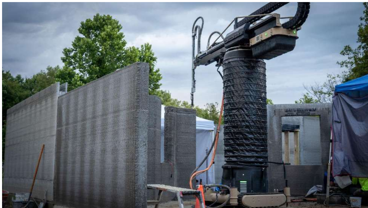
Slika 13 Sistem krana na gradilištu ( https://blog.apis-cor.com/the-effects-of-cement-and-global-warming-0 )
