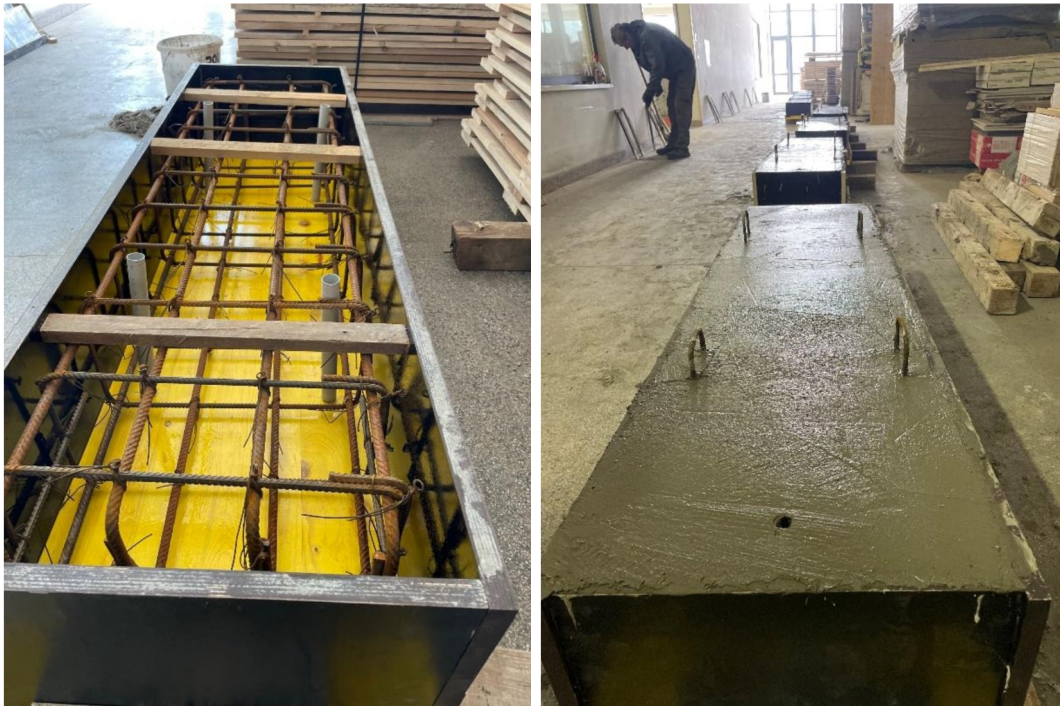
Figure 4.2 Formwork of the reinforced concrete beams
