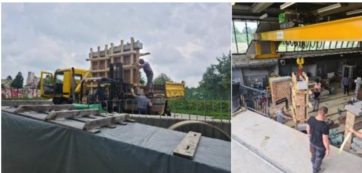
Figure 4.17 Transportation of masonry piers inside the laboratory
