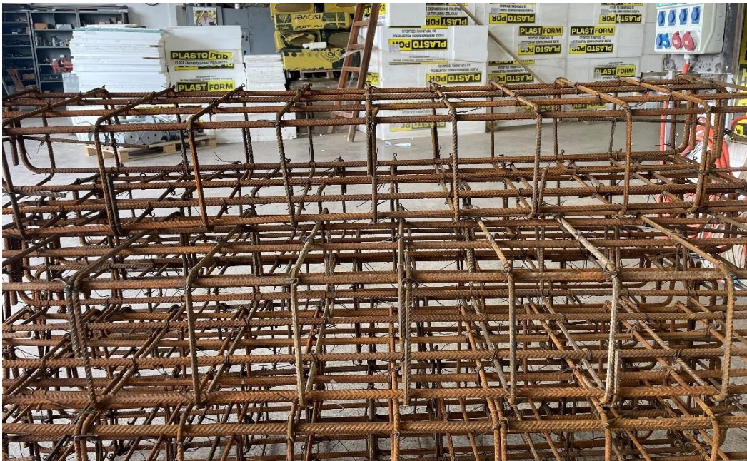
Figure 4.1 Construction of reinforcement cages
