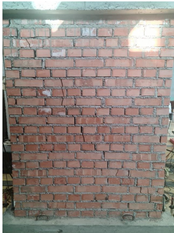
Figure 4.62 Final failure mechanism of CFRCM 3 pier
