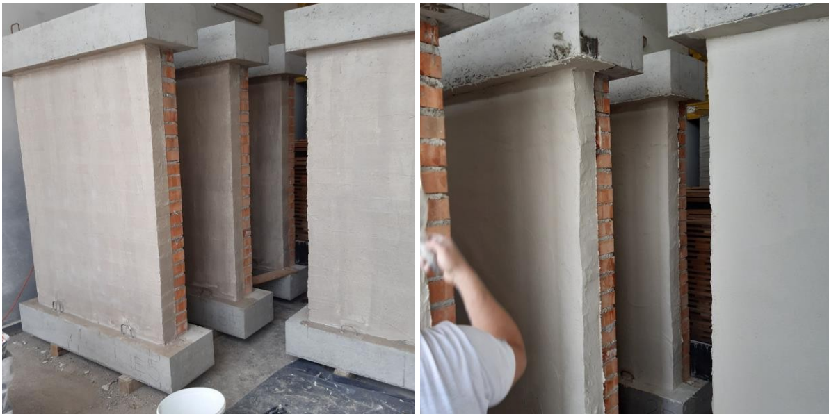
Figure 4.7 Strengthened masonry piers
