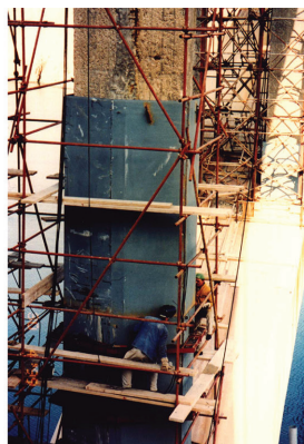
Figure 21. Strengthening of existing RC piers on Pag Arch Bridge in Croatia – cross section (left) and strengthening process (right) - (reproduced from [77])
