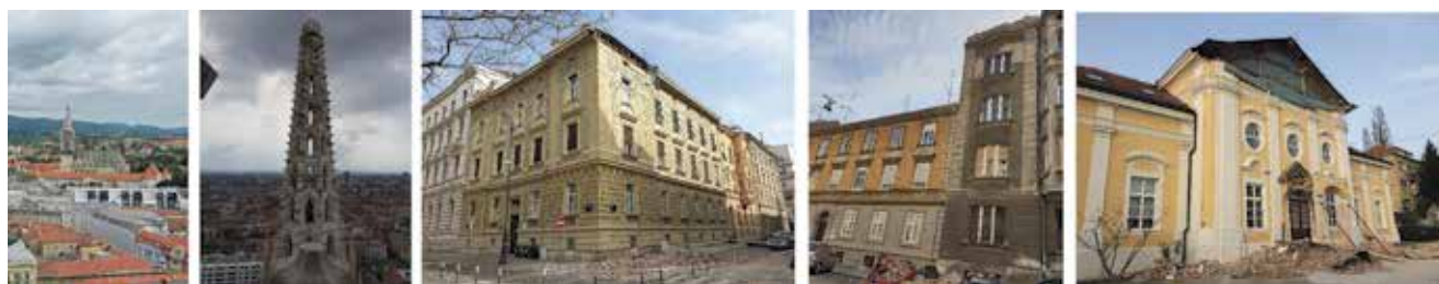
Figure 1. Earthquake effects in historic centre of the city (photos courtesy of: AIR-RMLD d.o.o. www.air-rmld.com , Filip Foretić, Karlo Jandrić)
