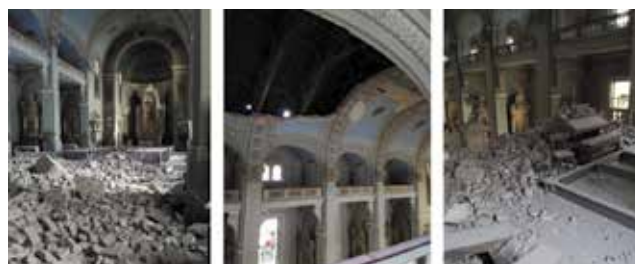
Figure 33. Damage to Basilica of the Sacred Heart of Jesus (photos courtesy of: Ivan Ćurić)
