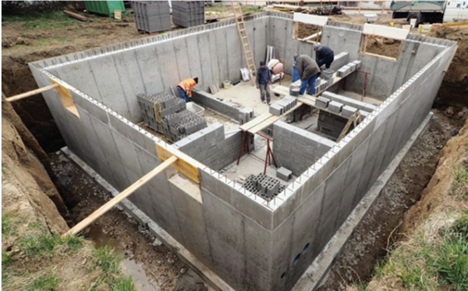
Figure 3. Commercial rigid basement construction
