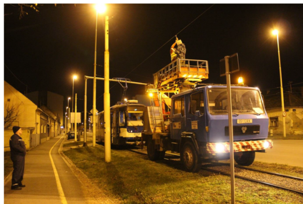
Fig. 3. Towing truck and tram T3 during overhead line measurements.
