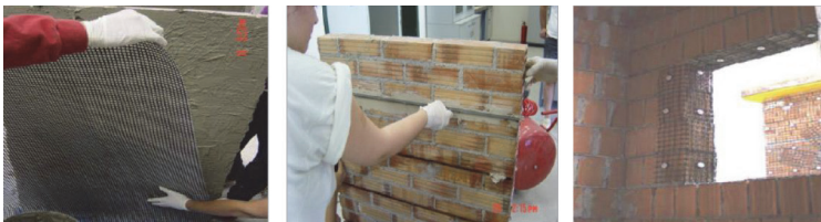
Figure 5. Use of FRP materials in restoration
