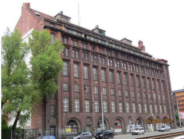
Figure 1: Current view of the flour warehouse
