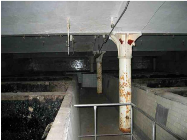
Figure 11: RC reservoirs with cast iron columns
