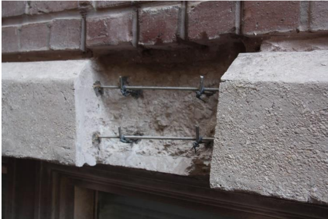
Figure 3: Installed stainless steel rods in edge of slab
