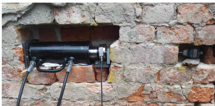
Figure 5: Shear test, building 7 – outside wall
