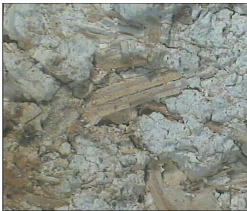
Figure 4a: Straw in the structure of old lime mortar
