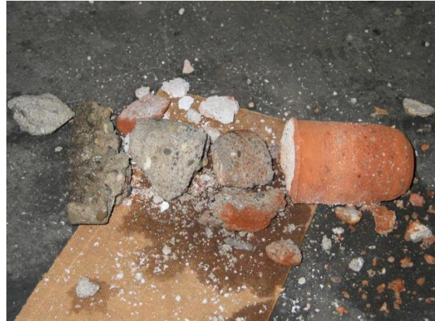
Figure 16: Drilling core of stables floor
