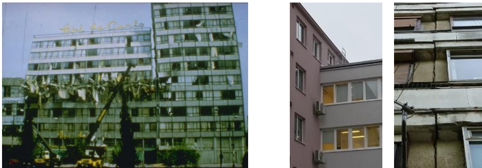
Figure 1: a) Examples of pounding effect during an earthquake [2]; b) photographs of separation gaps in analysed examples
