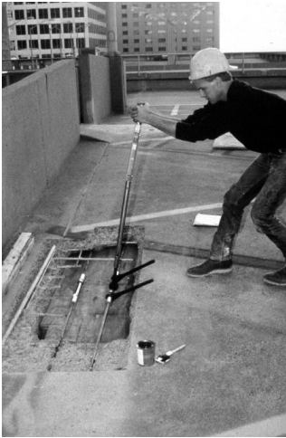
Figure 14: Calibrated torque wrench
