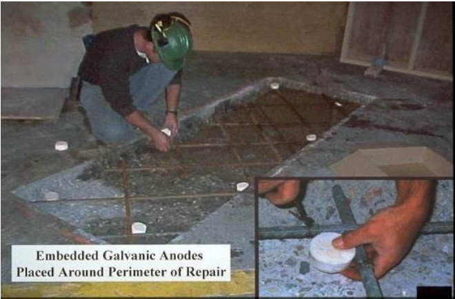
Figure 4: Installation of galvanic corrosion anodes
