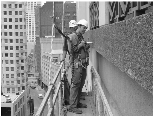
Figure 15: Impact echo test of facade panels
