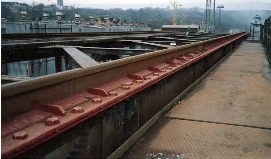
Figure 4: Top chord of semi-gantry crane girder after repair
