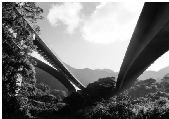
Figure 8: View from below of a post-tensioned cast-in-place box girder bridge
