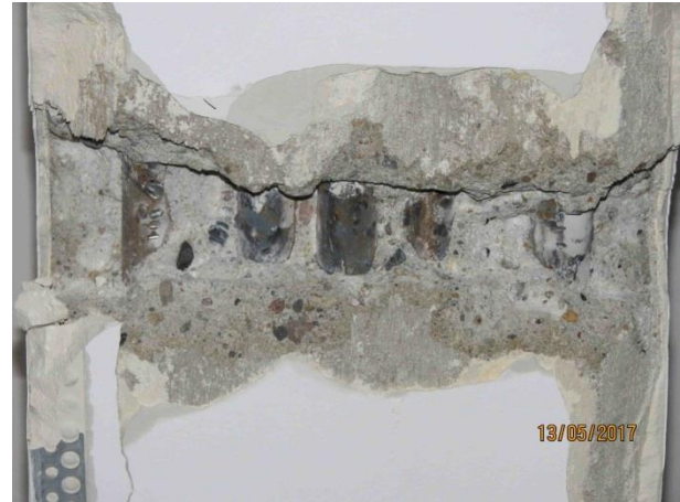
Figure 4: Reinforcement identification
