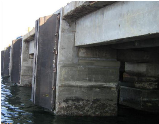
(c) Piers after repair (with rectangular cross-section)
