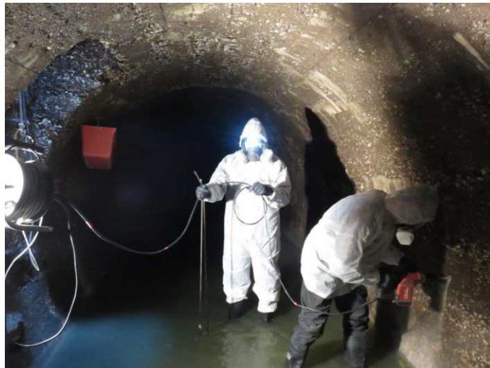
Figure 3: Work conditions inside the sewerage pipe
