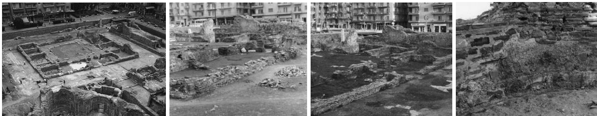
Fig. 1-4 Preservation state of the Galerius Palace after the intervention of the 70's [1]
