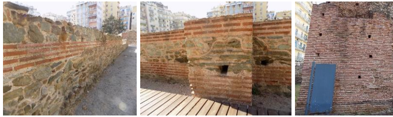
Figure 8 Preservation state of the complex's masonries 20 years after repair
