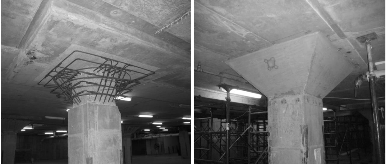
Figure 4: Column capital prior to and after concrete placement
