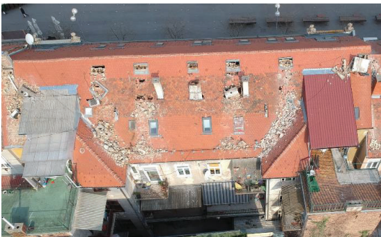
Figure 6: Timber roof collapse – Sisak cathedral (photo credit: Studio Arhing d.o.o.)
